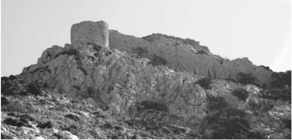
The second and latest phase of the fortifications at Kastro Apalirou seen from below.
